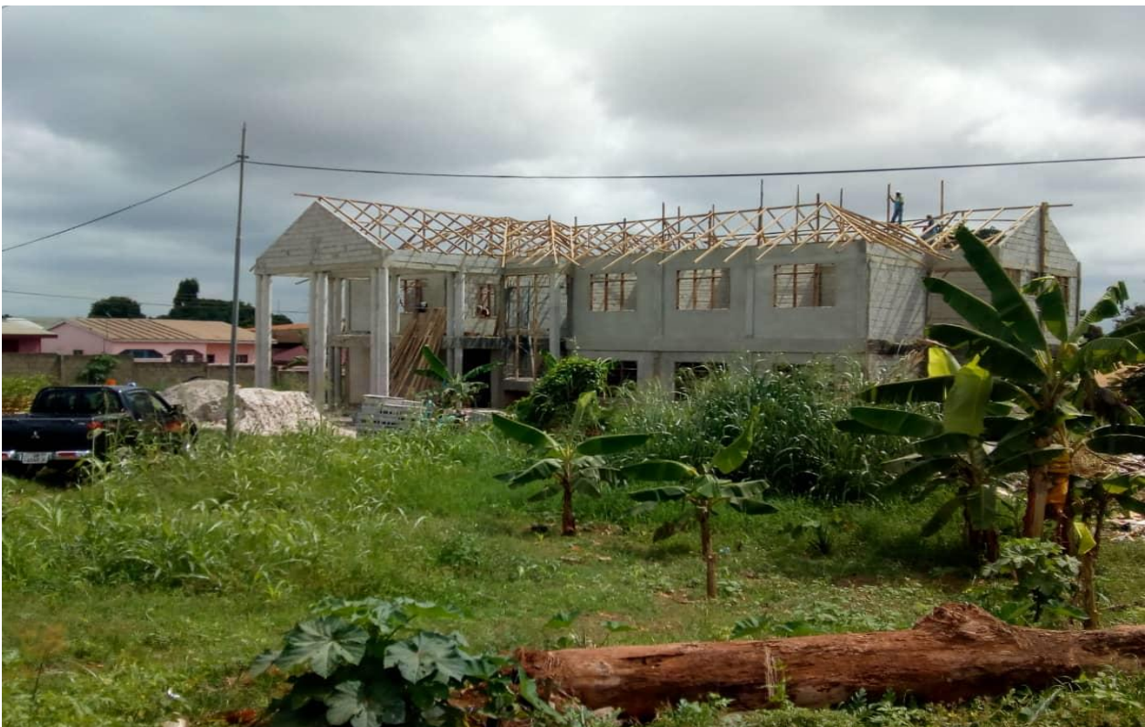
Figure 11: Ongoing construction of Nhyiaeso Sub-Metro Office at Fankyenebra.
