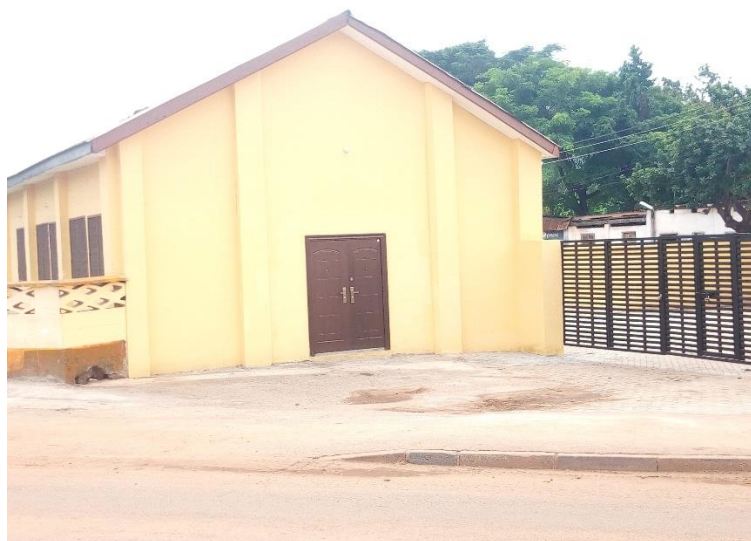
Figure 3: Rehabilitated Circuit Court Building At Adum
