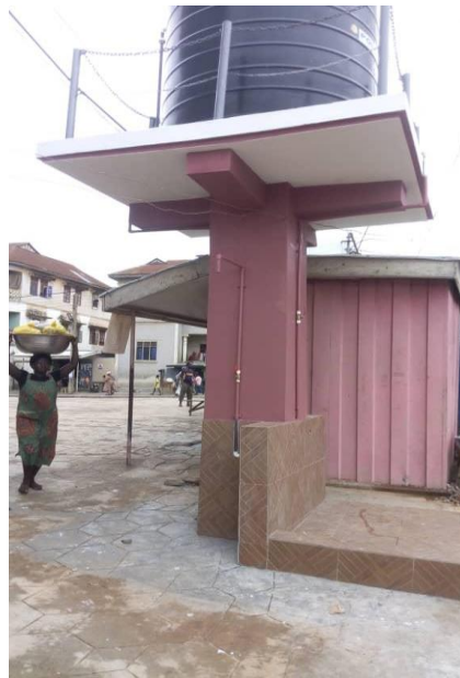
Figure 5: Mechanized Borehole With An Overhead Tank at Bohyen
